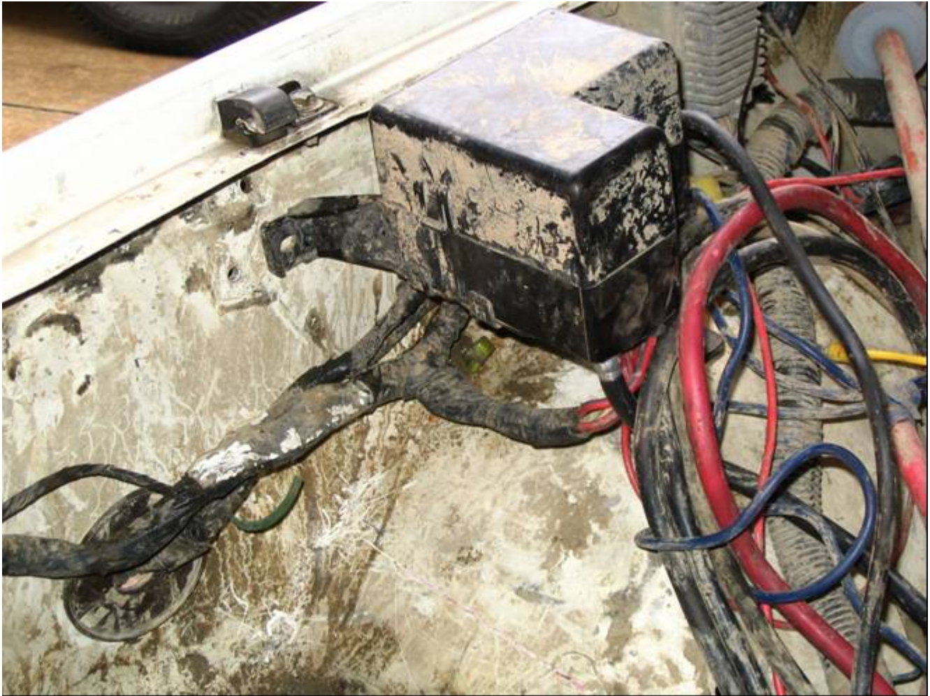
Figure 2. OEM fuse box moved to the rear approximately 1". The wiring harness visible to the left has just enough play to allow this movement without rewiring.
